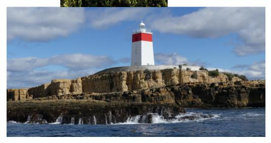
Built of curved cast iron pieces in 1906, Tasman is the highest operating lighthouse in Australia at 276m above sea level. It was converted to wind power in 1975, automated in 1976, and the station demanned in 1977. It is not open to climb, but we're free to photograph it and view memorabilia displayed in keepers' cottages.
